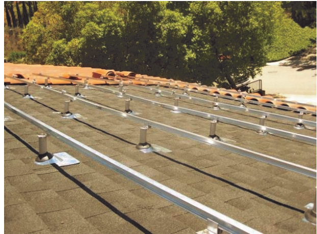
Figure 2.5: Standoff mounting system for roof top (several inches off the roof surface allowing natural venting) Source: Unirac
