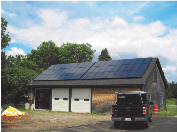
Figure 2.4 Integral rooftop mounting system (attach directly to roof rafters) at the Boston Nature Center.
